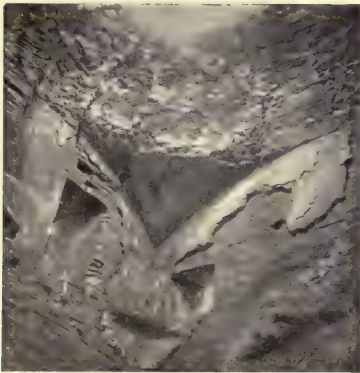
Fig. 47.—Rome. Tomb on the Via Nomentana. Pendentive of Dome (II nd Century).
